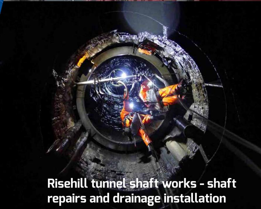
Risehill tunnel shaft works - shaft repairs and drainage installation
