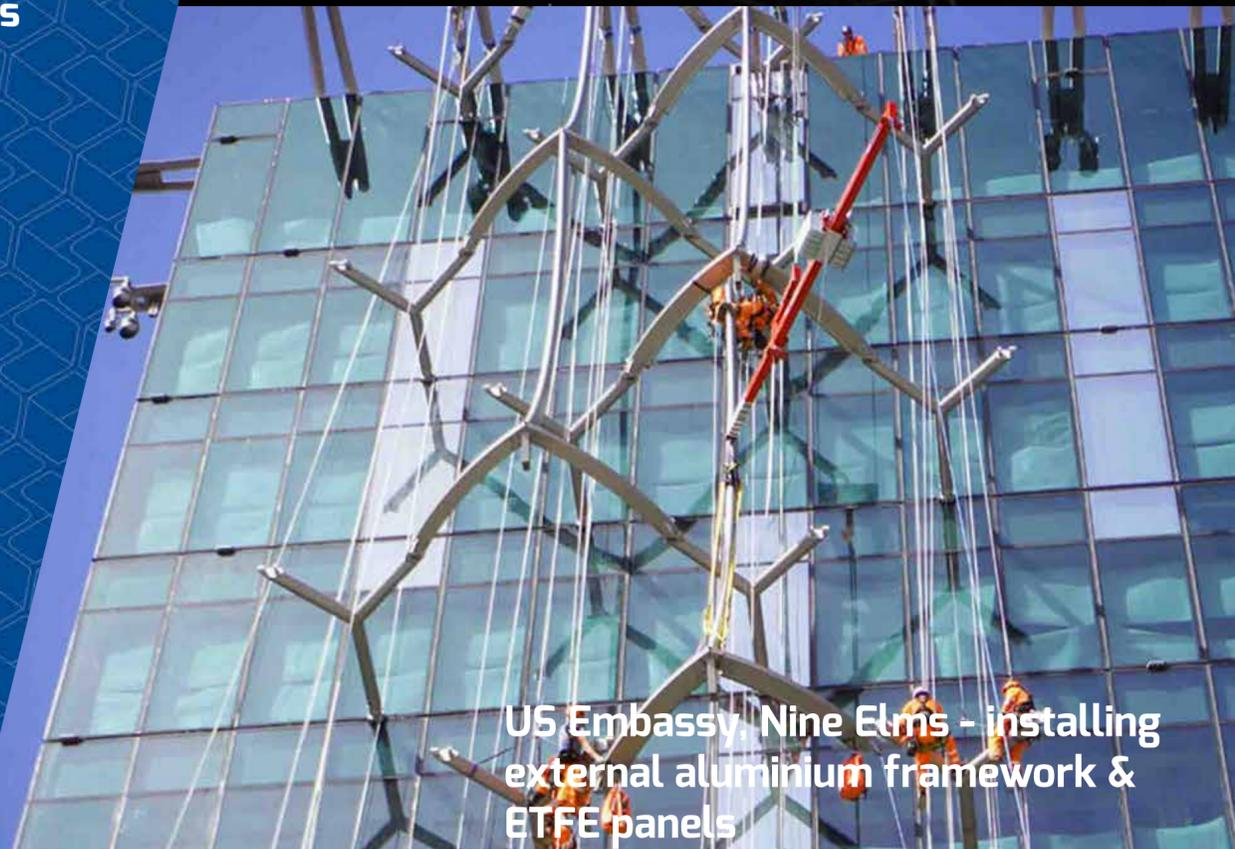
US Embassy, Nine Elms - installing external aluminium framework & ETFE panels
