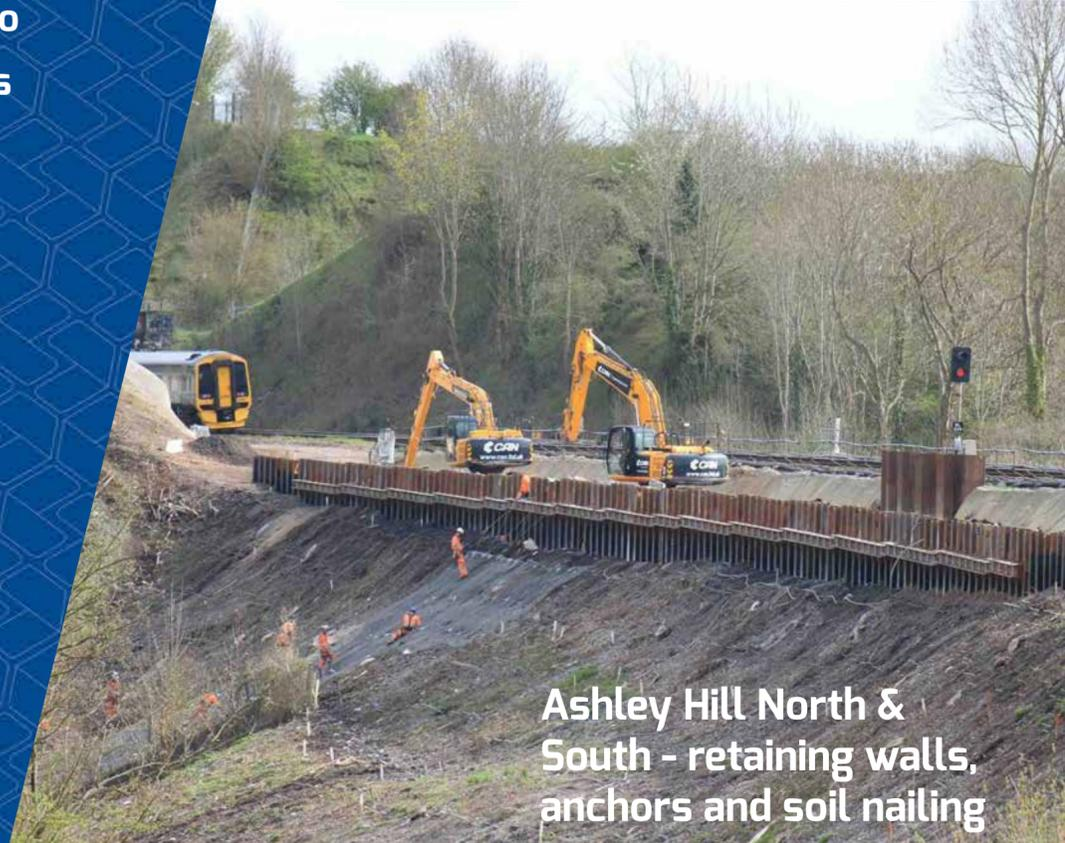
Ashley Hill North & South - retaining walls, anchors and soil nailing
