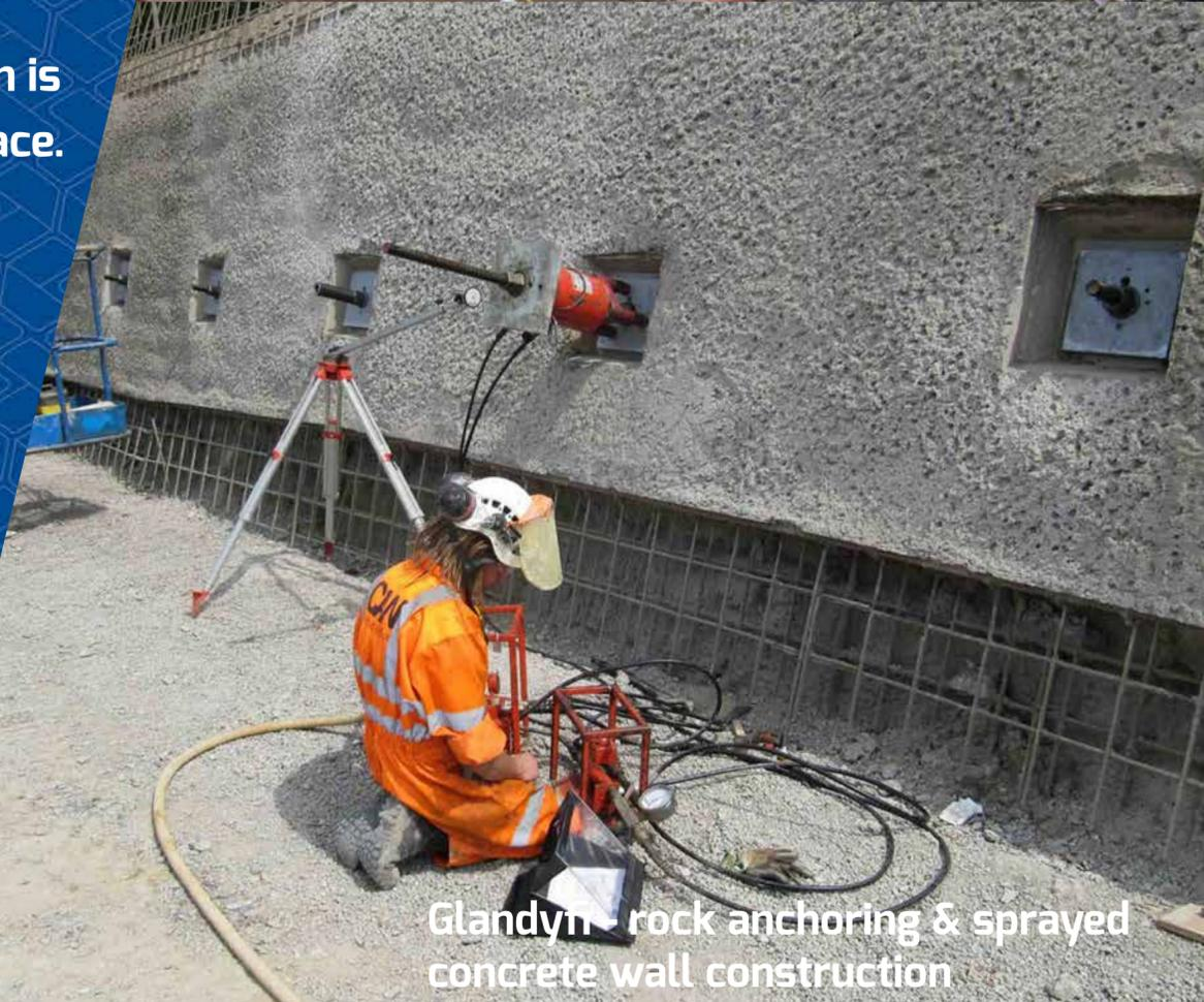
Glandyn - rock anchoring & sprayed concrete wall construction
